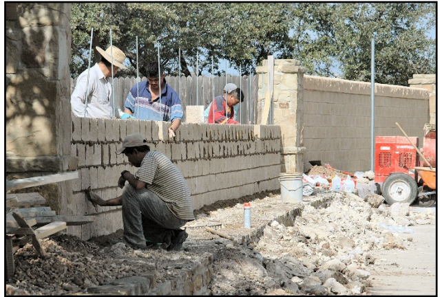
Construction crew building roadway wall
