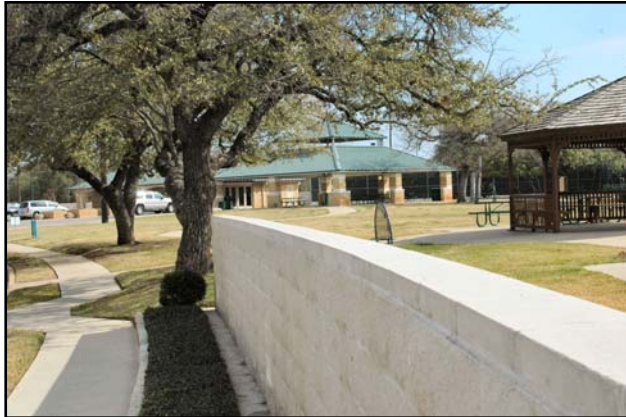
Neighborhood street view with retaining wall (Old Mill Road looking from Gazebo toward District office)
