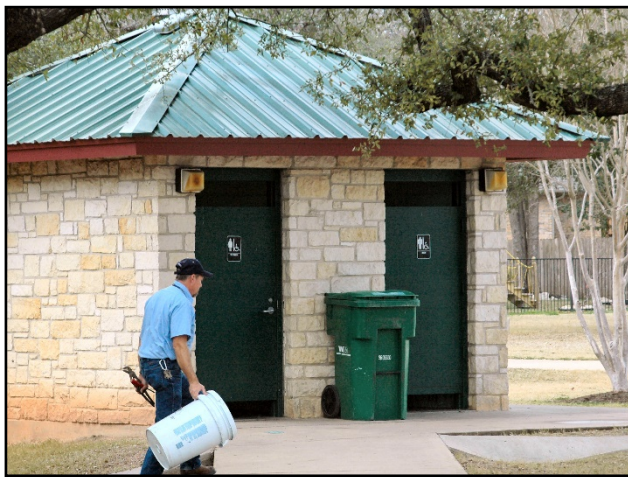
Neighborhood park restroom maintenance
