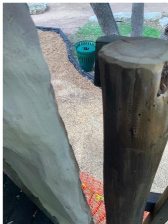
The length and width of the engineer wood fiber is non-compliant with ASTM.
