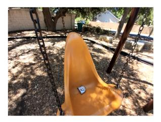
Compliant 12.6.6. Swing hangers are spaced wider than seats, not less than 20". (ASTM 8.6.1.5)
